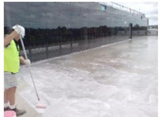
Figure 1 Applying epoxy primer
