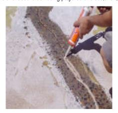
Flexural Cracking: These cracks are caused by engineered design structural faults and will readily sheer most membranes. In proper design, expansion joints stress relievers are inserted in the area where a flexural crack will develop (engineers can calculate this). In these circumstances, the application of Ultra Flex is suitable.
