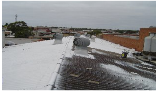
Encapsulating asbestos sheeting with Heat Block
