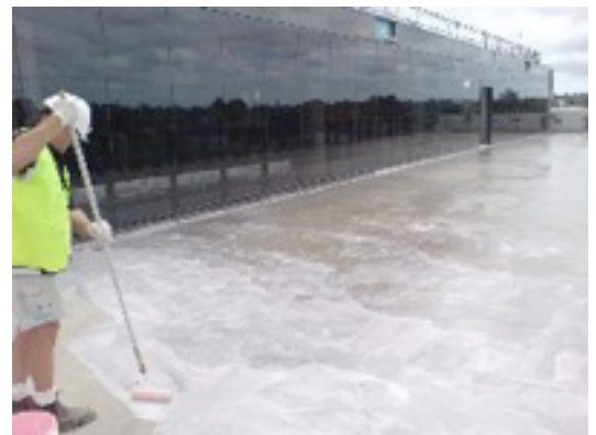
Figure 1 Applying epoxy primer
