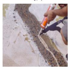
Flexural Cracking: These cracks are caused by engineered design structural faults and will readily sheer most membranes. In proper design, expansion joints stress relievers are inserted in the area where a flexural crack will develop (engineers can calculate this). In these circumstances, the application of Ultra Flex is suitable.
